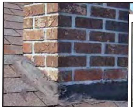
*Chimney with cracked and deteriorated flashing*
